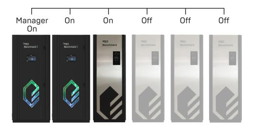
**Reduce Emissions:** Prioritize the electric boiler to reduce building emissions while using gas to cover design load days
